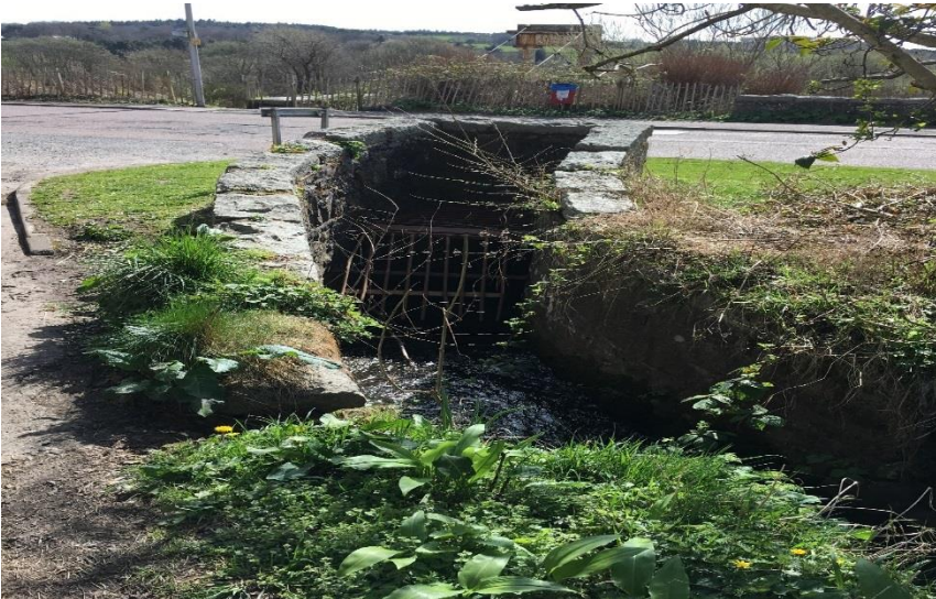
Figure 6: Burn of Cults Culvert Inlet
