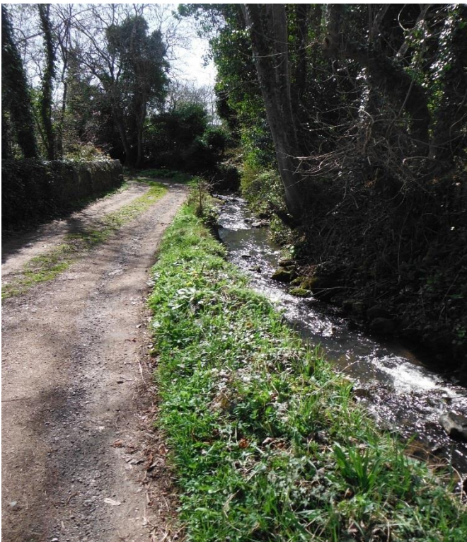
Figure 13: Burn of Cults Open Channel
